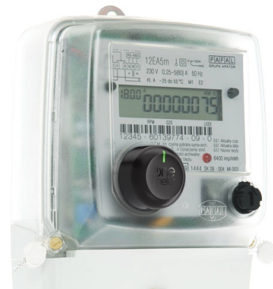
Figure 1. OneMeter beacon with optical sensor attached to IEC 62056-21 port of electricity meter.
