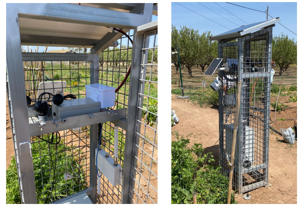
Figure 2. System deployed in anti-vandalism enclosure.
