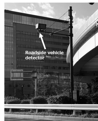
Fig. 1. Roadside vehicle detector.
