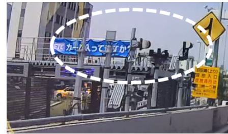
Fig. 9. Roadside vehicle detector.
