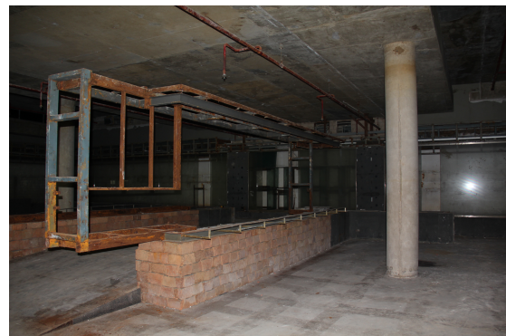
Figure 3. SEACM was seriously affected from the worst flooding in Thailand 2011.
