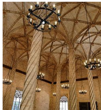
Figure 1. This pilot experiment took place in the room of columns at the Silk Exchange, Valencia. This room is the most charismatic space in the building and it characterised by its slender twisted columns.
