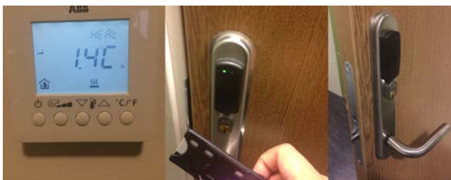
Figure 3. Heating control (left) and RFID door (right)
