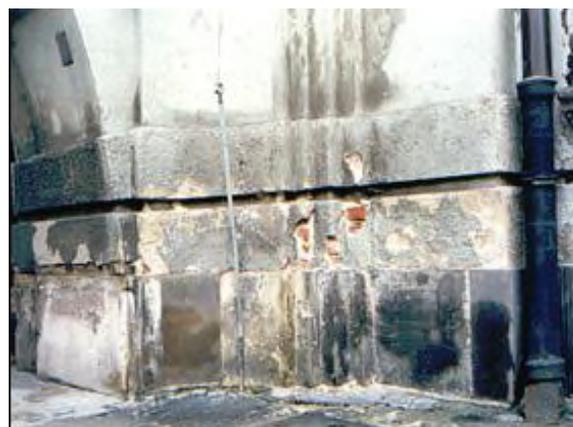
Figure 1. Historical damp wall. Examples of excessively damp brick walls in historical buildings.
