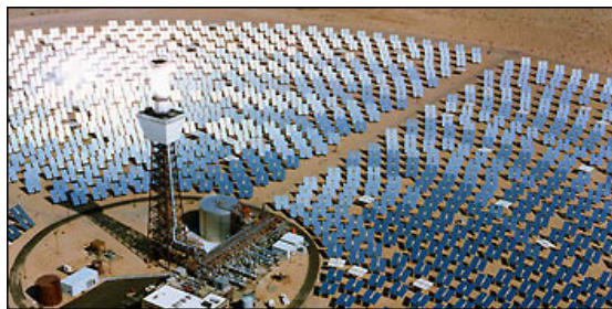
Fig. 9. Solar Two Power Plant (Wikimedia Commons License).
