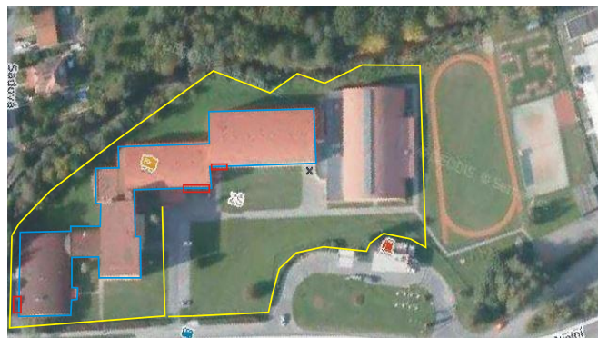
Figure 7. Technical security of large school.
