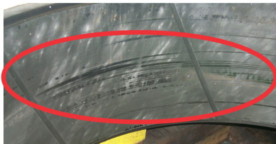
Figure 2. Photography of a damaged bearing that is disassembled to perform corrective maintenance.
