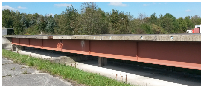
Figure 1. This figure shows the bridge for our tests.
