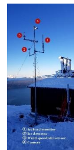
Figure 2. The installed weather station at Linken Narvik
