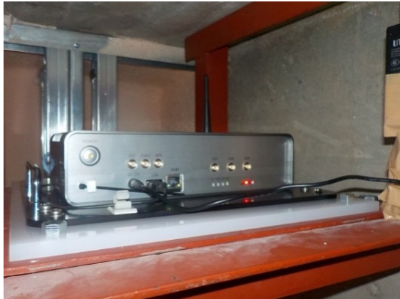
(a) Ceiling of 3 rd floor (Floor of rooftop)
