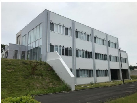
Figure 6. External appearance of building.
