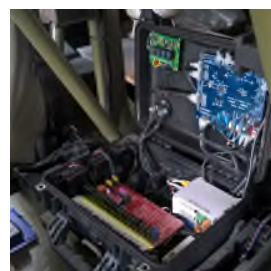
Figure 4. Electronic and communication control box
