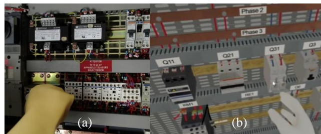
Figure 2 : Actual electrical cabinet (a) and associated VR modelling (b)
